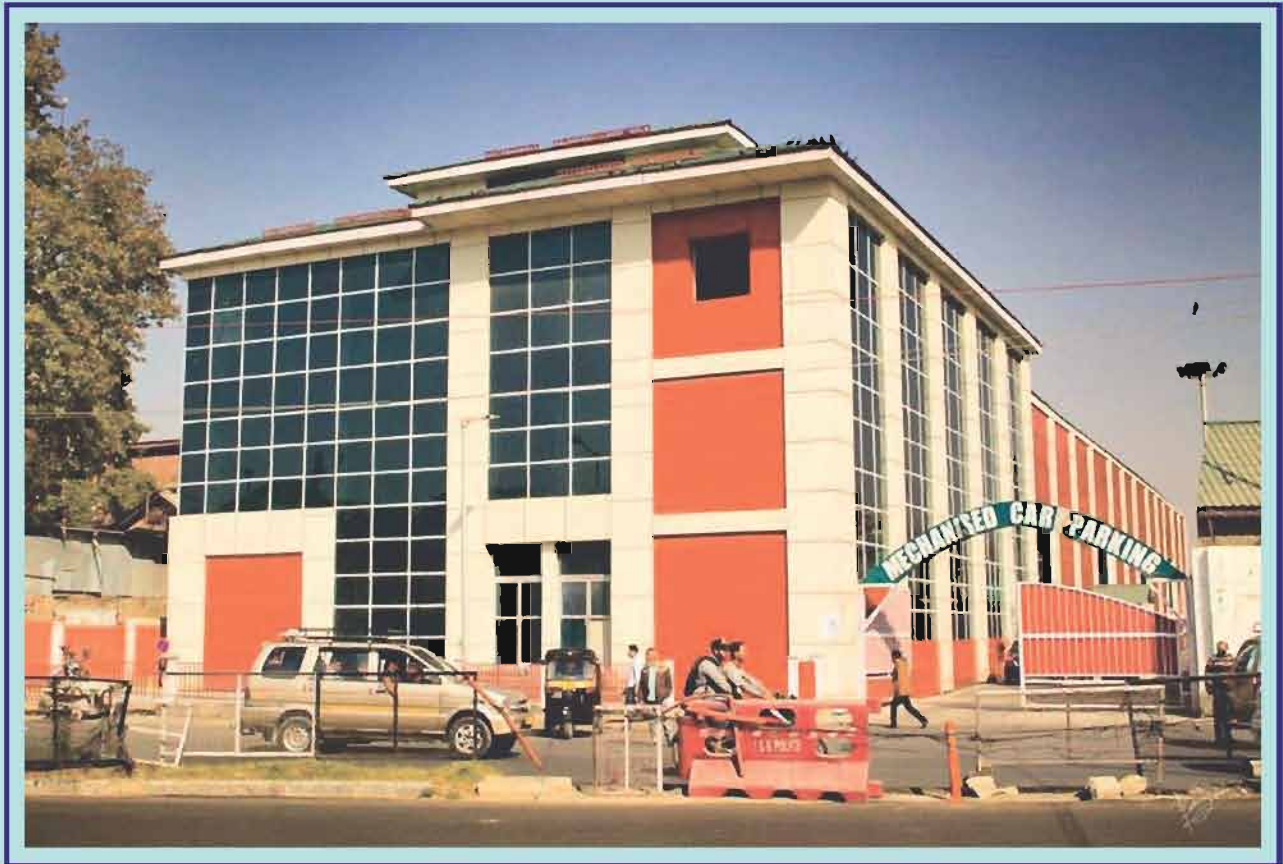
MECHANISED CAR PARKING, Srinagar
